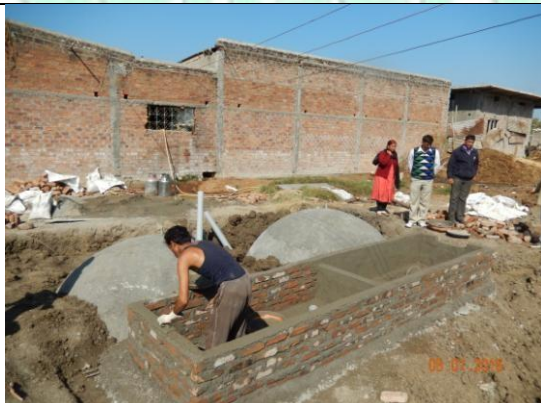
Construction of bio gas plant
