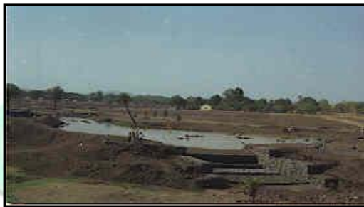
Gabion as outlet of water harvesting tank at College campus
