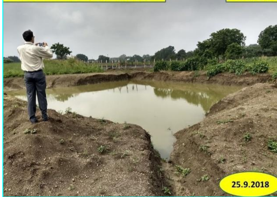
Percolation tank and lined water harvesting tank INDORE 2018
