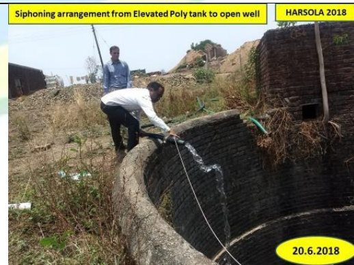
Siphoning arrangement from Elevated Poly tank to open well HARSOLA 2018
