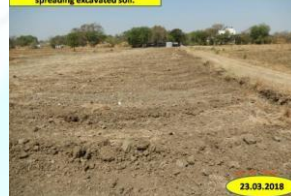
Newly created cultivated field after spreading excavated soil. INDORE 2018
