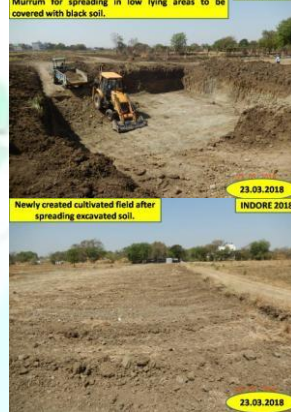
Newly developed percolation tank - excavated Murrum for spreading in low lying areas to be covered with black soil. INDORE 2018
