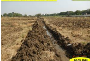
Leakage from pipe diverted through drain INDORE 2018
