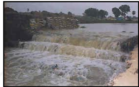
Gabion as outlet of water harvesting tank at College campus
